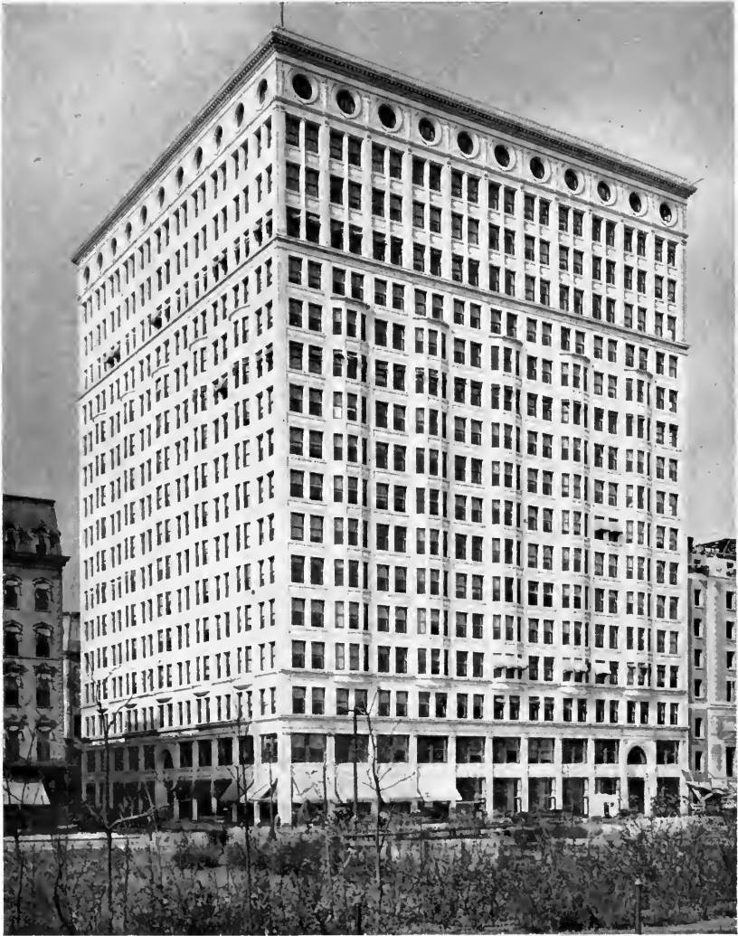
THE RAILWAY EXCHANGE BUILDING, CHICAGO, ILL.
